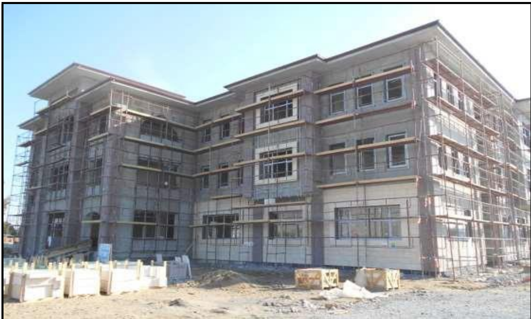
Figure 117 Construction of Yamantürk Vocational College, January 2017
