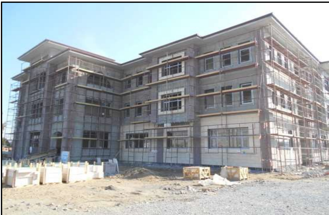
Figure 117 Construction of Yamantürk Vocational High School, January 2017
