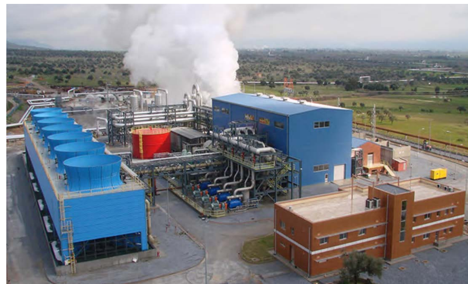
Figure 1–The existing Gürmat GPP
